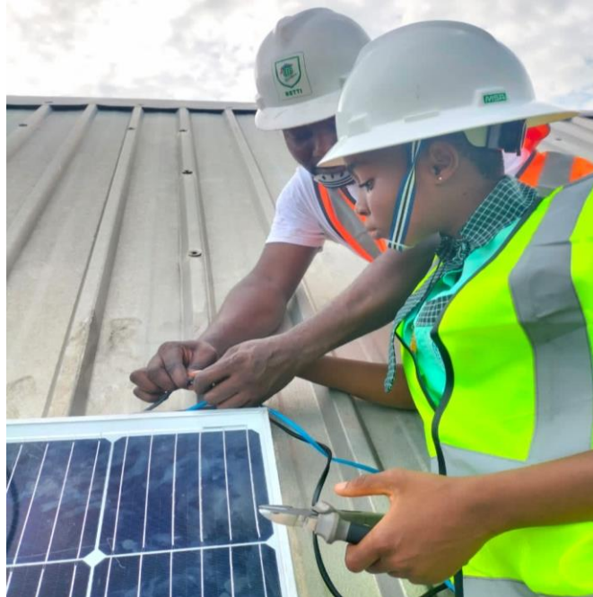
Student participating during solar installation at rooftop
