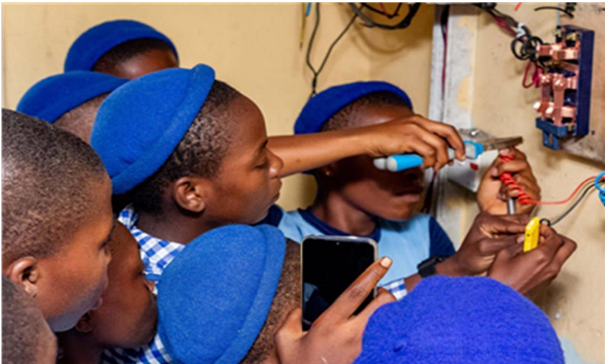
Students installing a change over system
