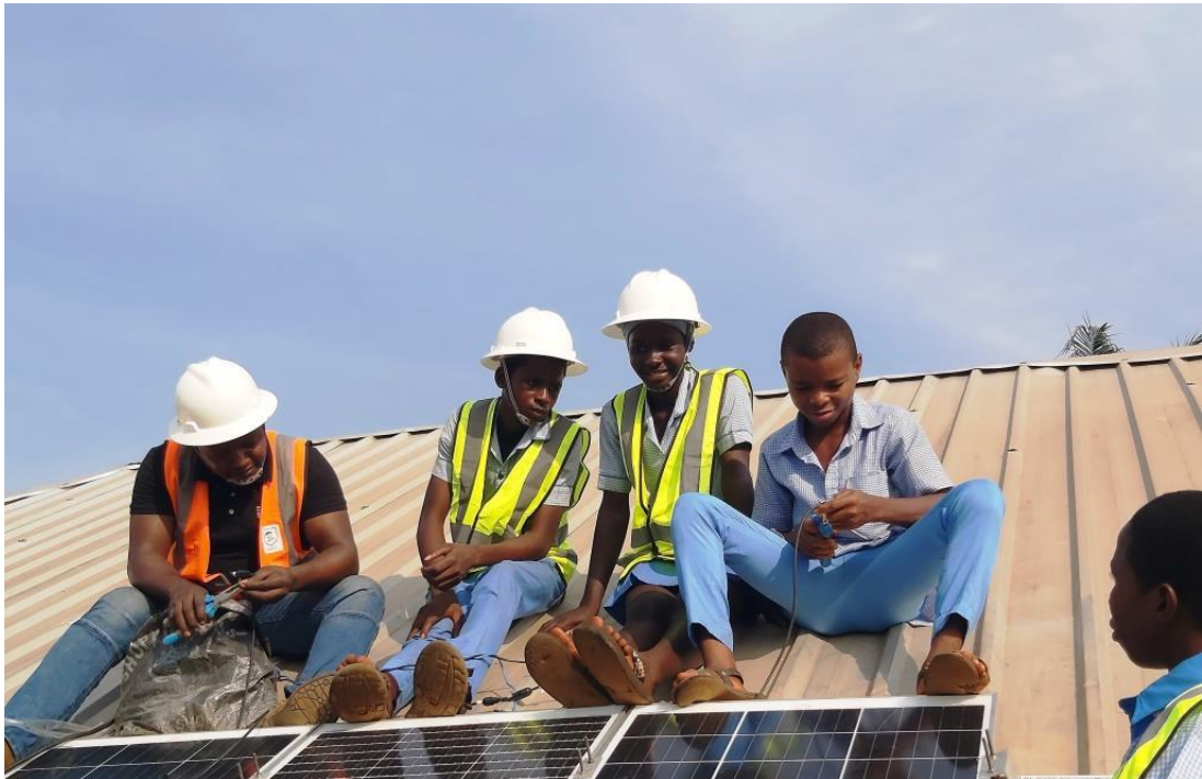
Trainees installing a solar panel at a roof top
