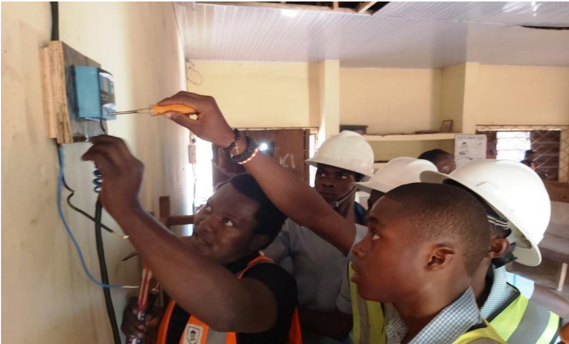
Trainees learn how to install a charge controller
