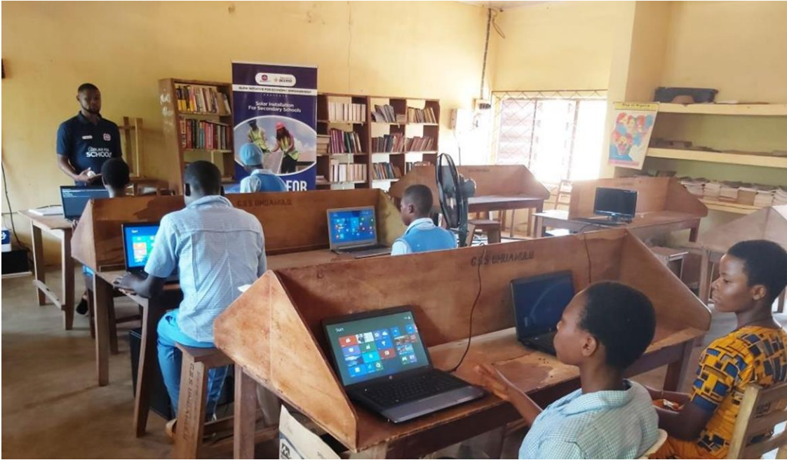
Students power their computer systems after the solar installation
