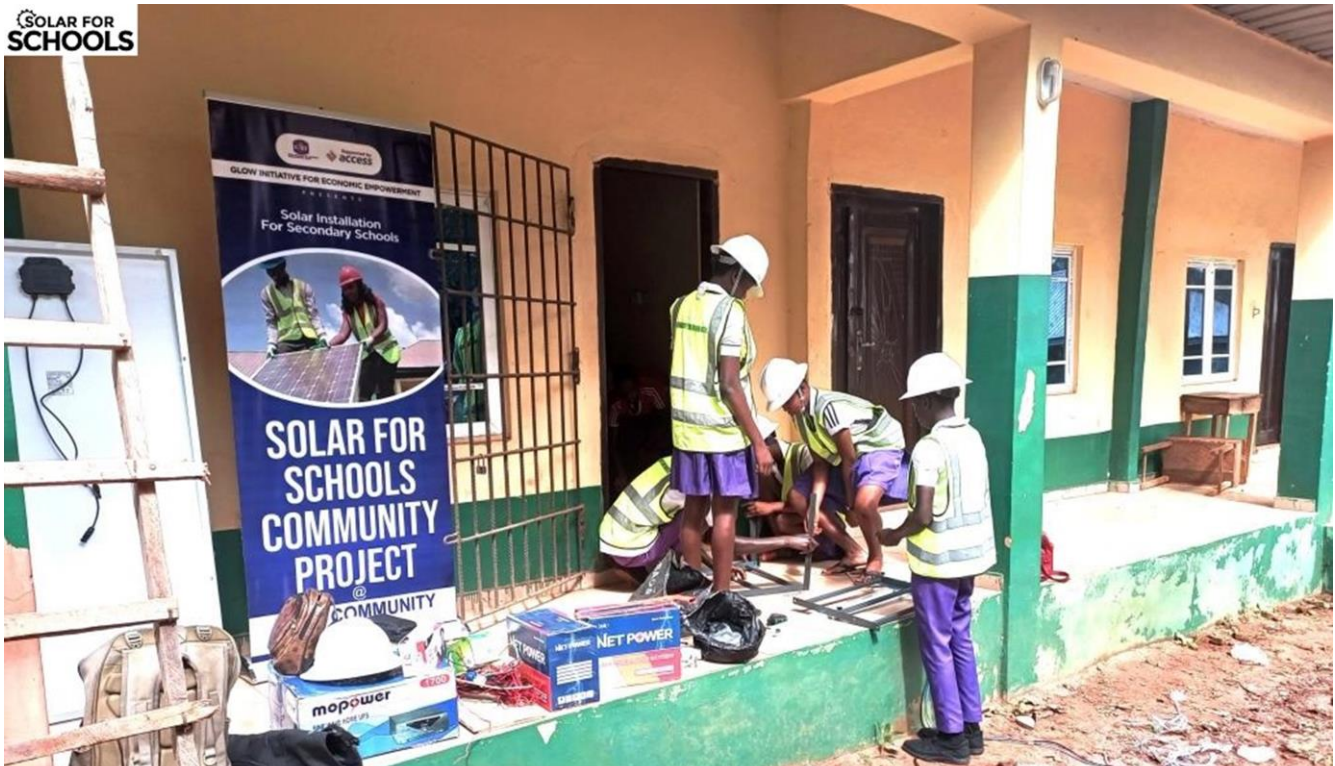
Students coupling a rack during the installation
