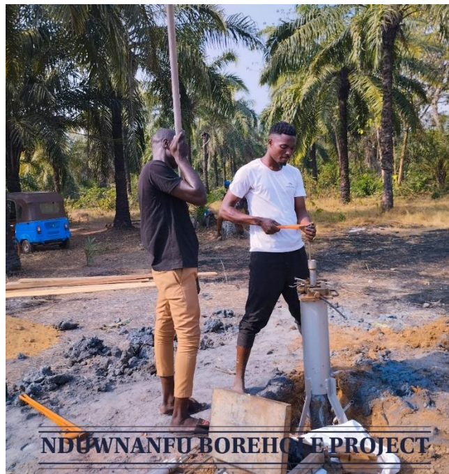
The installer during the installation process on the drilled site.
