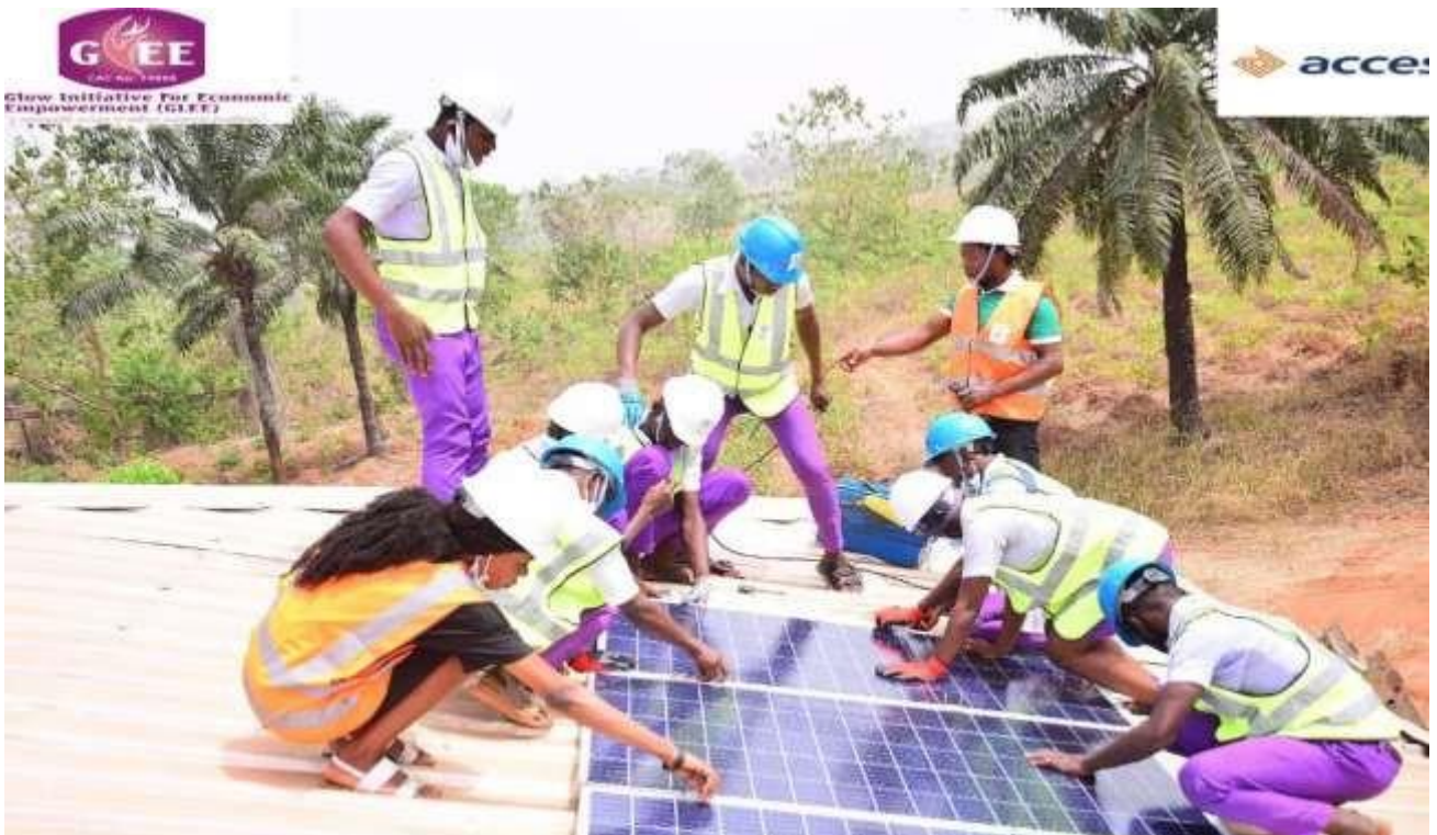
Students learning and participating in the solar installation process
