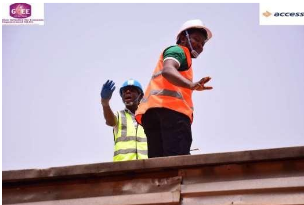
At a roof-top for solar panel installation
