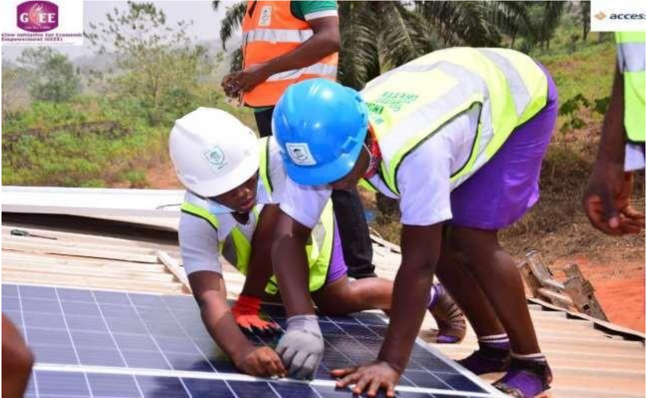
Two female students on a roof top screwing a bolt on a solar panel
