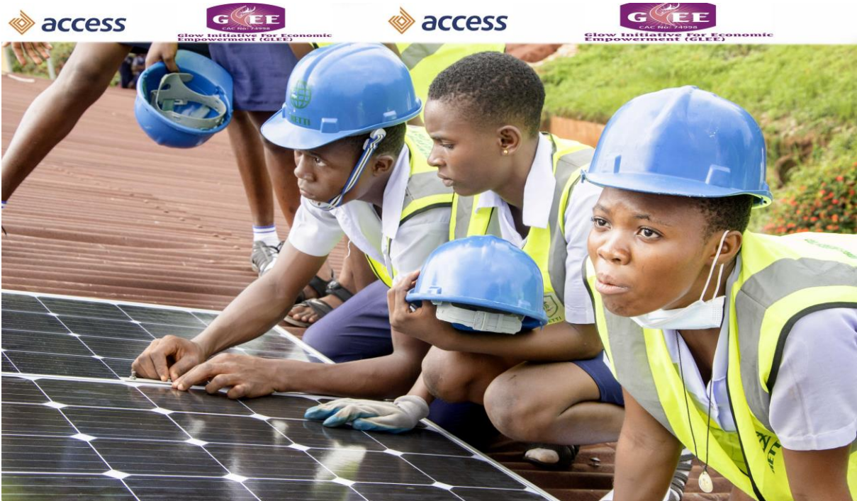
Students installing solar panels at a roof top
